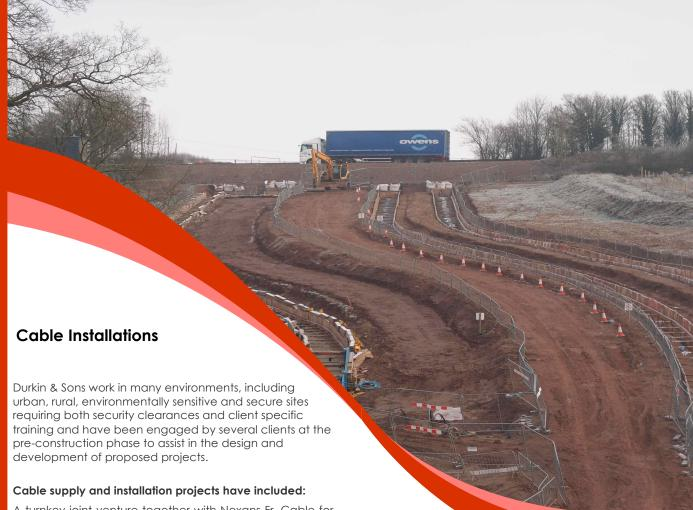
A turnkey joint venture together with Nexans Fr. Cable for EDF Energy at West Burton power station, Nottinghamshire. Works consist of the design, supply and installation of cable network, route length of 1,800 metres between the new switchyard of the new power station and National Grid switch room of 400kV single circuit. Ducted installation.
